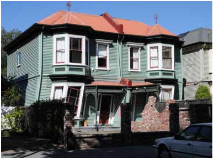
This turn-of-the-century wooden residence in Christchurch New Zealand was moved off its foundation during a 6.3 magnitude earthquake in 2011.
